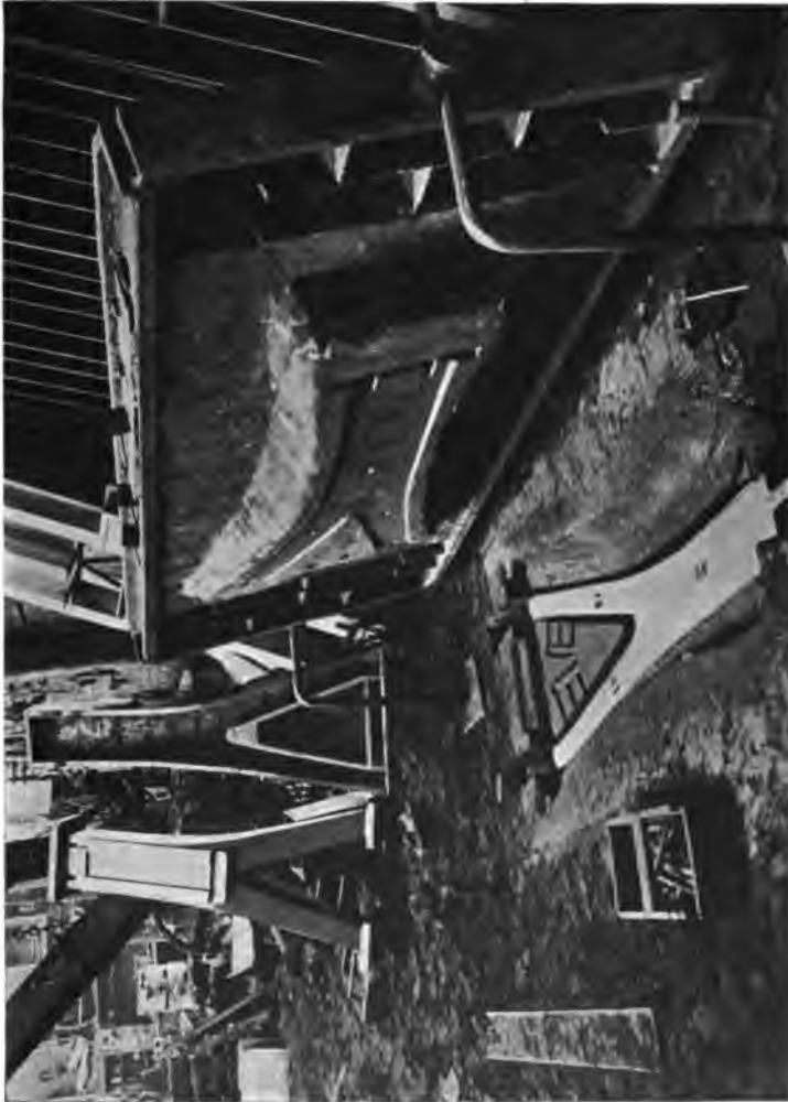
FIG. 187.—Back Standard for Inverted Vertical Engine. Mould with Cores in Position.
